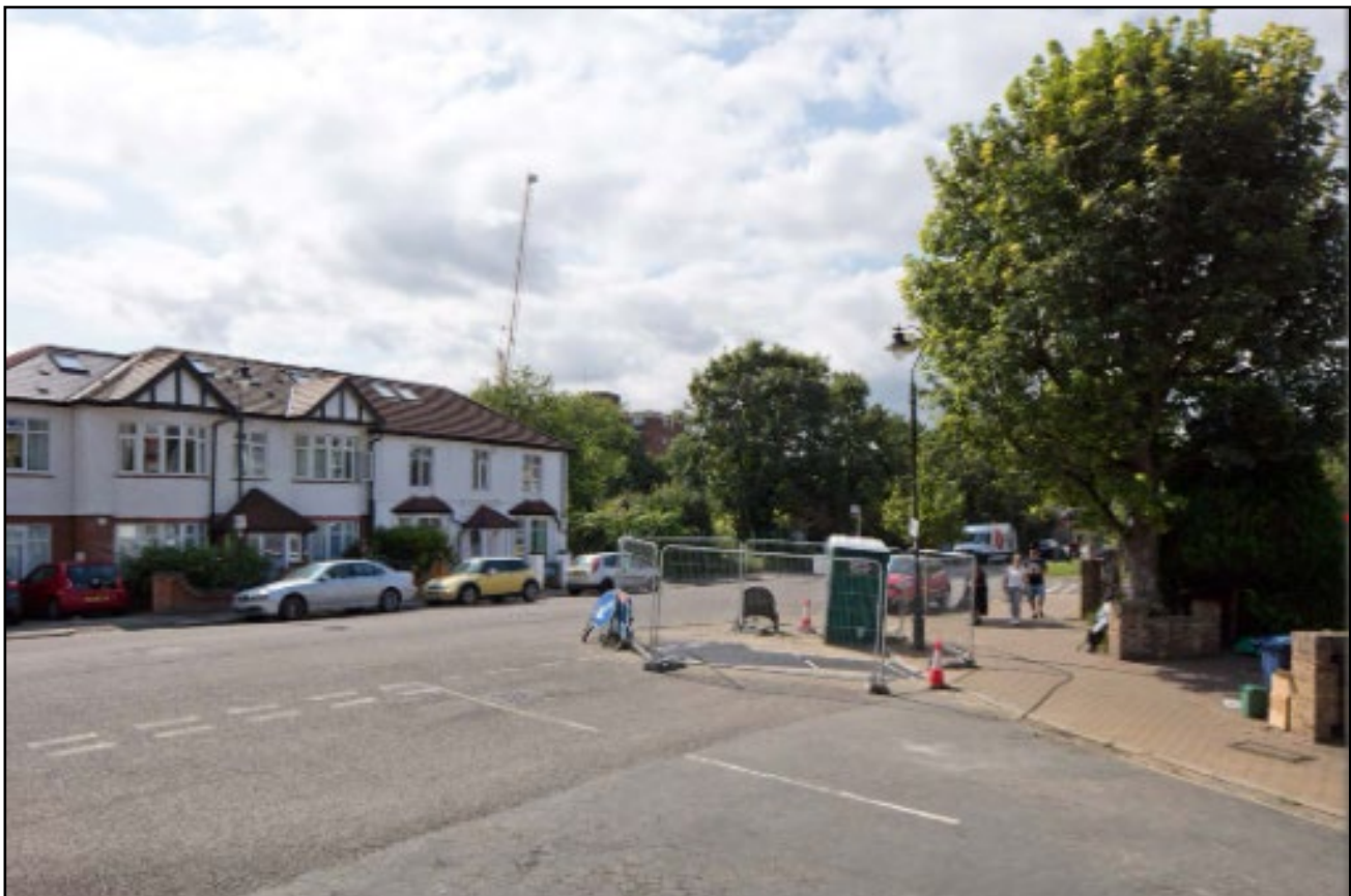
Figure 13: Existing View from Mattock Lane
